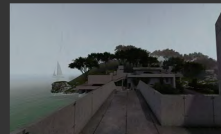
Exit from the auditorium, concrete bridge link to the service building which sitting on the rock and covered with plants.
